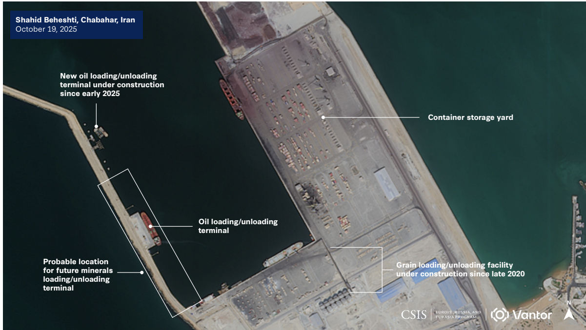
Figure 5b: New Oil Loading and Unloading Terminal, Shahid Beheshti Port, Under Construction in 2025
