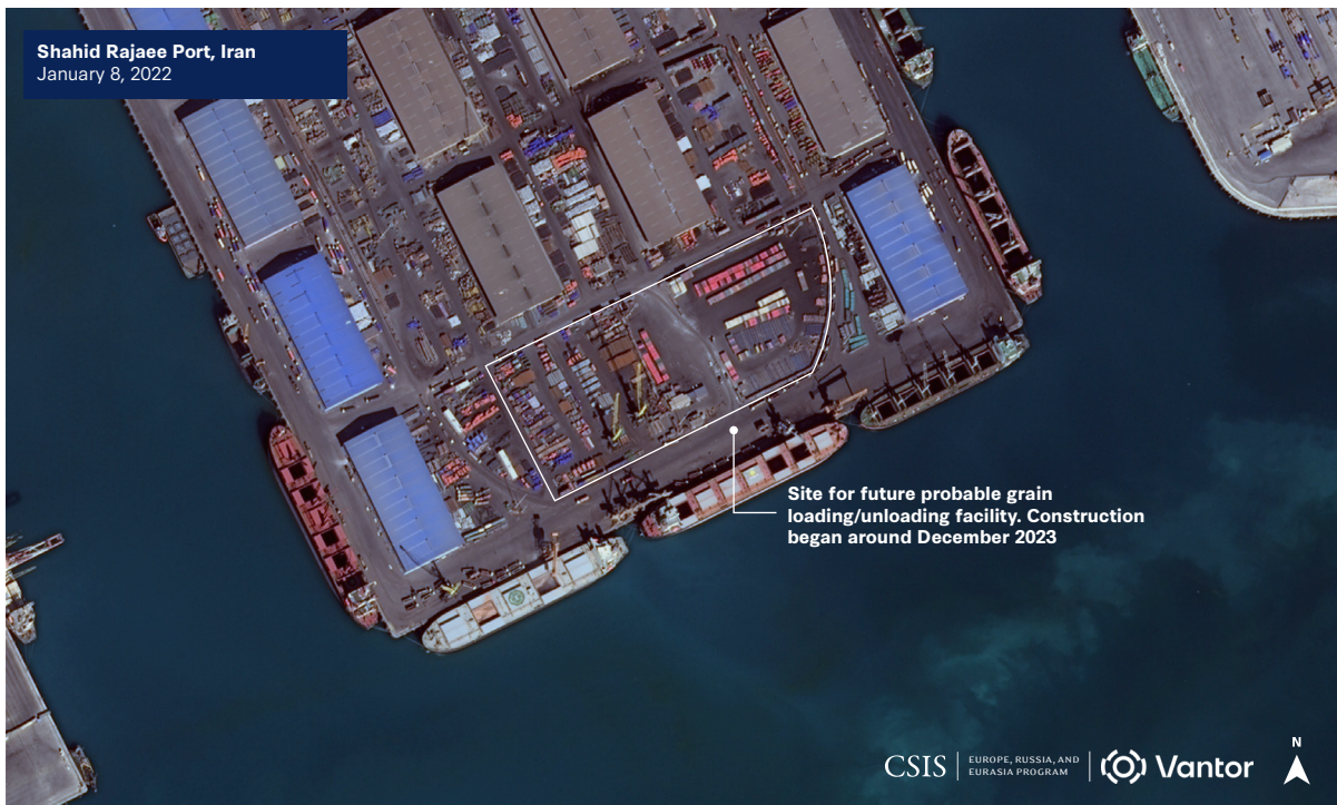
Figure 4a: Probable Grain Loading and Unloading Facility, Shahid Rajaei Port, 2022
