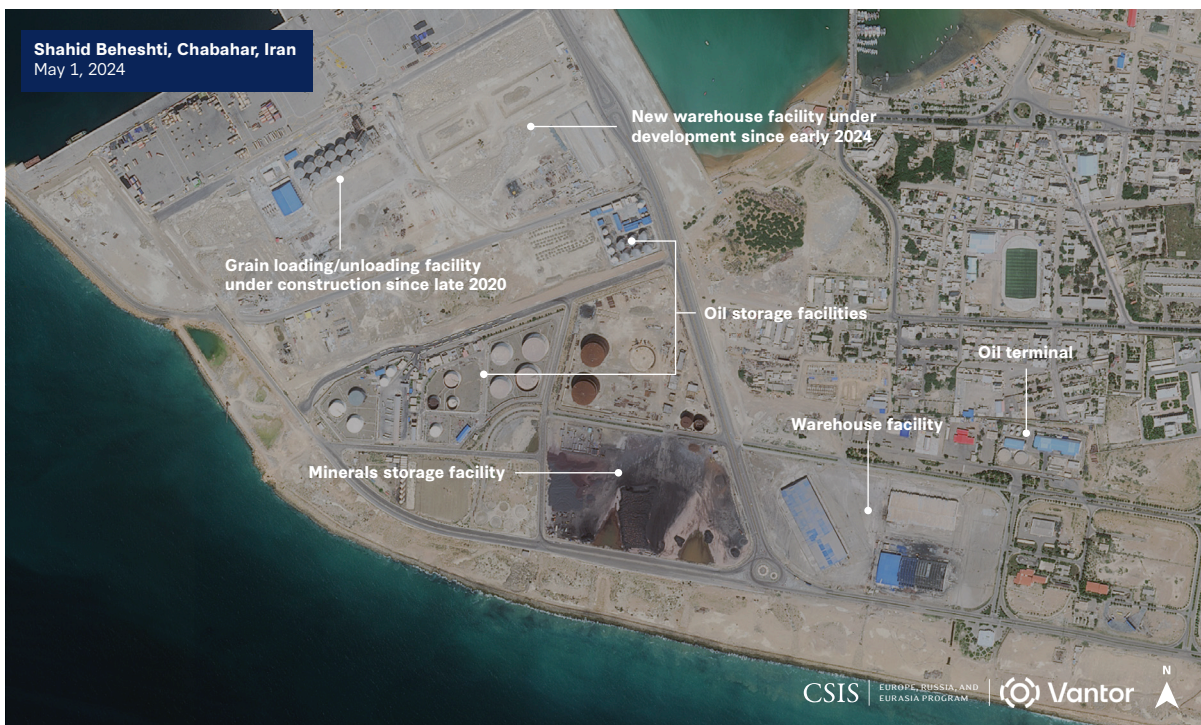
Figure 6a: New Warehouse Facility, Shahid Beheshti Port, Under Development in 2024
